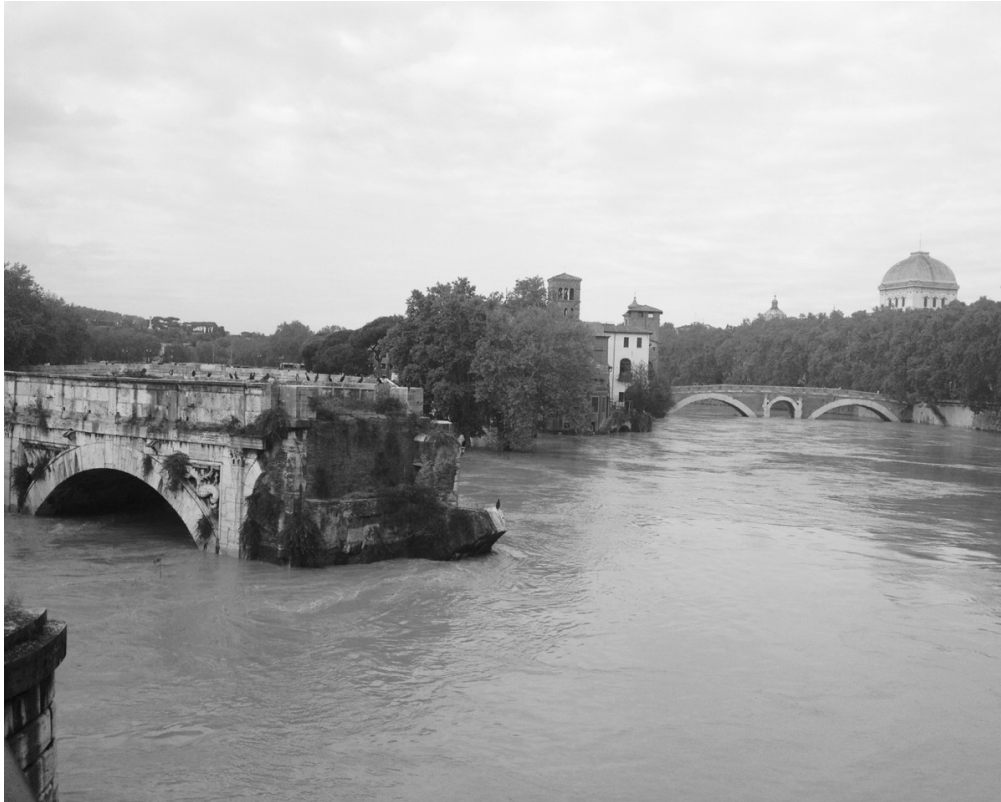
Ponte Rotto and the Tiber island during the 2012 floods
